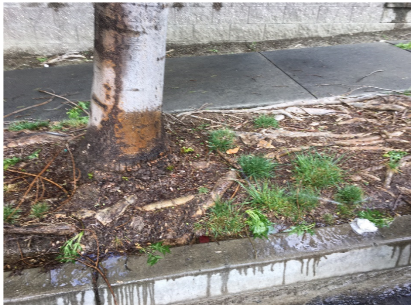
Photo 7. An ash tree that has inundated the planting strip, broken the irrigation and is clearly too large for the space allotted.
