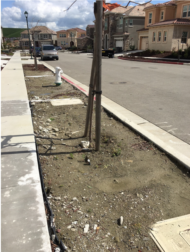
Photo 8. Trees planted in Dougherty Valley in the spring of 2017. The soils are compacted and construction debris is present.
